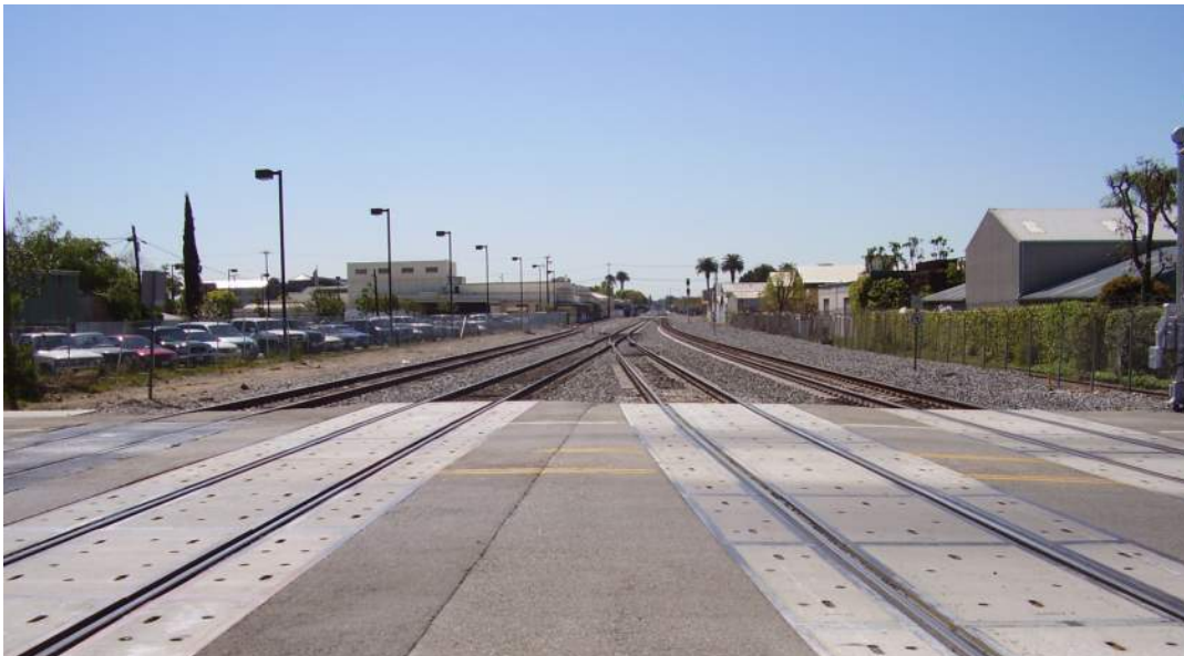
Figure 3-38. Location of Turnout Adjacent to Highway-Rail Grade Crossing
