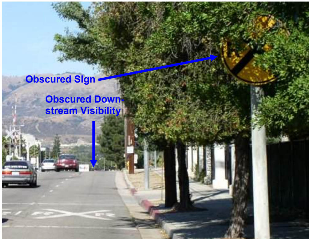
Figure 3-15. Restricted Visibility at a Highway-Rail Grade Crossing Approach
