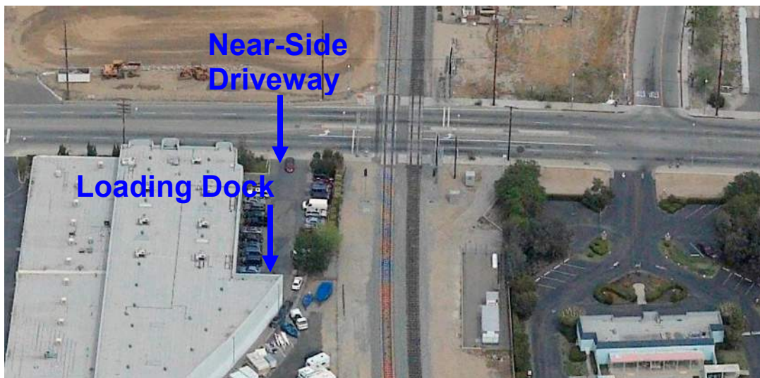
Figure 3-14. Loading Dock Adjacent to Right-of-Way
