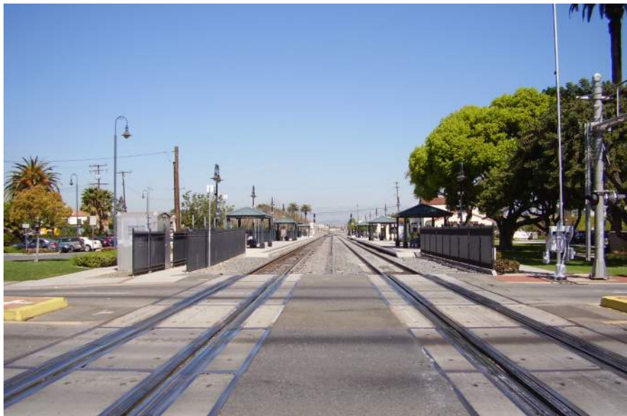
Figure 3-35. Stations near a Highway-Rail Grade Crossing
