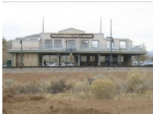
Photo 3: Main Shelter (Train Side View)
