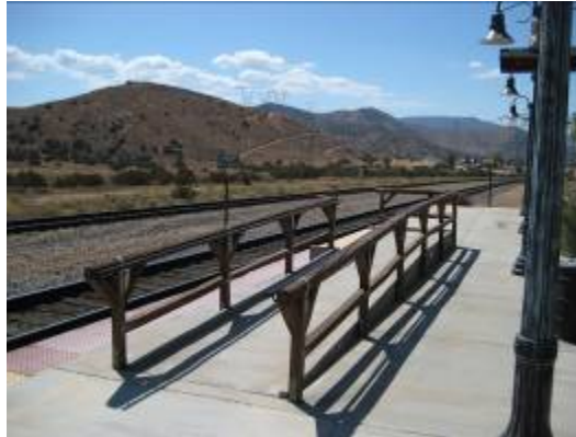
Photo 1: Existing ADA Mini-Platform Ramp
