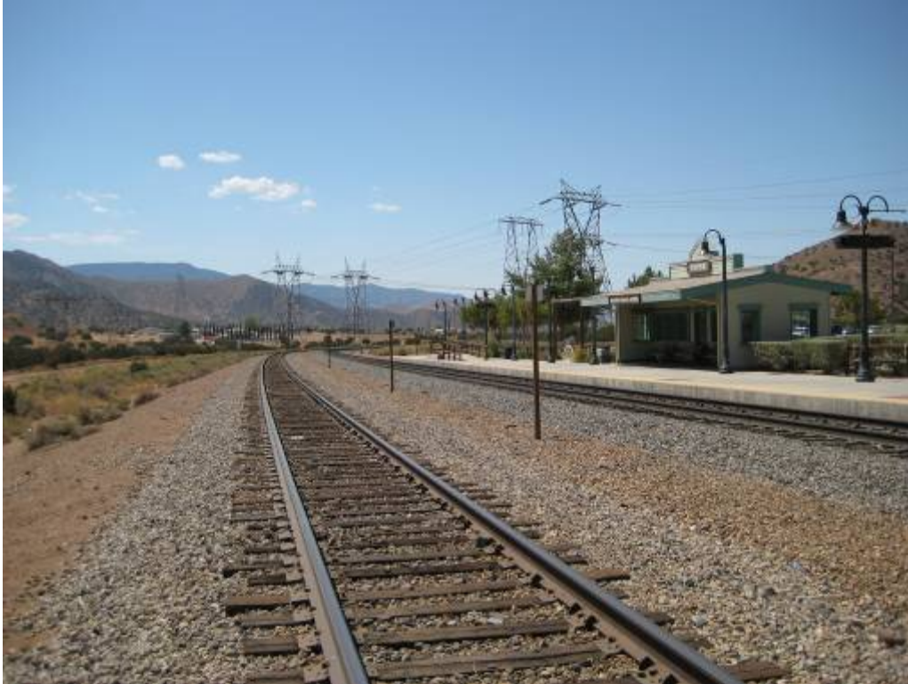
Southwest facing view (view toward LA Union Station) Pictured: (Left to Right) Subject Site, Vincent Siding, Mainline Track, Existing Platform
