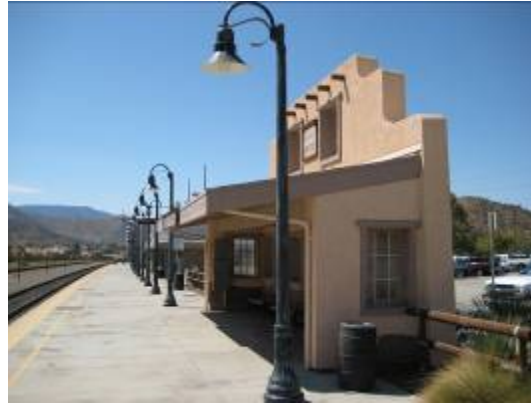
Photo 5: "HOTEL" Shelter (Train Side View)
