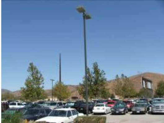
Photo 12: Parking Lot Area Lighting
